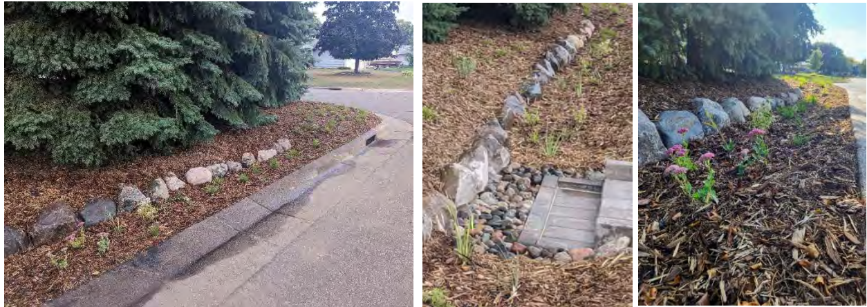
[Above] Forster curb-cut bioretention, Lily Lake subwatershed.
